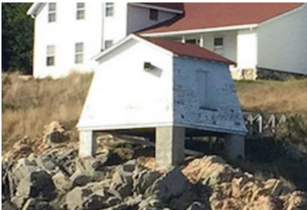
This is the Bell House from the South East Side. The Lichen is apparent on both the south and east sides of the building.
